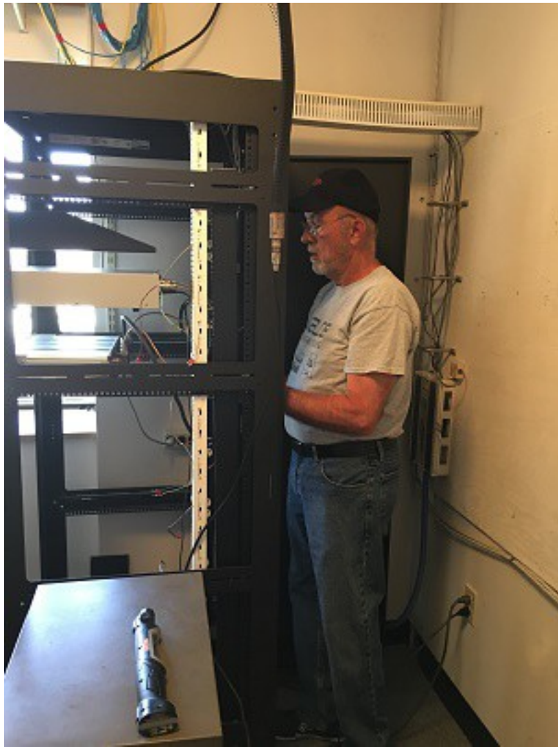
Jack (KC9KY) working on the repeater.
